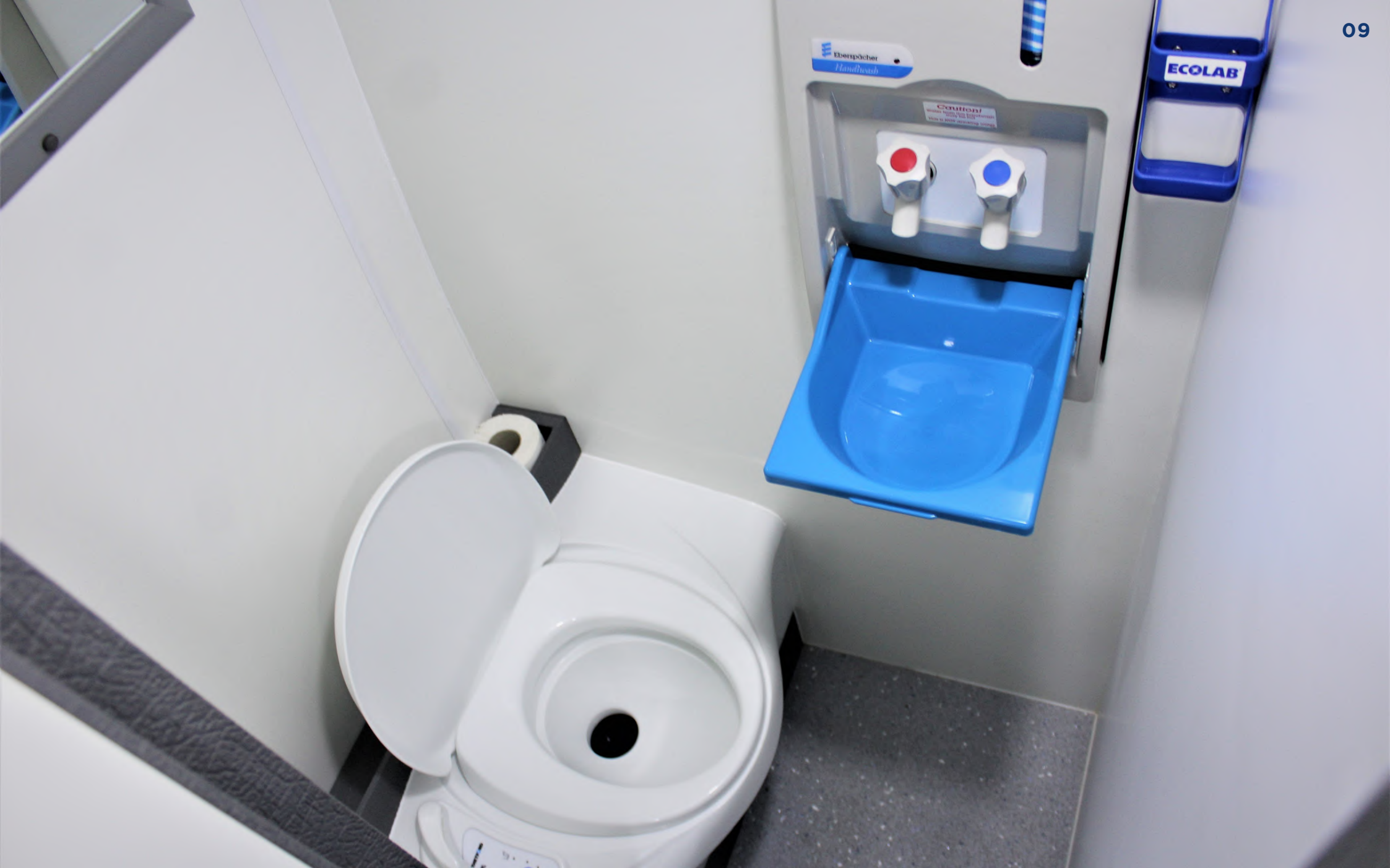
WASHROOM WITH TOILET & HOT / COLD WATER SINK
